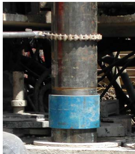
Photo courtesy of K&K Well Drilling - Batavia
