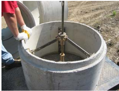
lifting concrete casing
