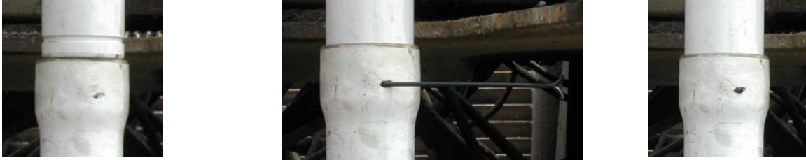
Photos courtesy of K&K Well Drilling - Batavia
