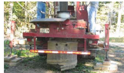
ready to start boring
