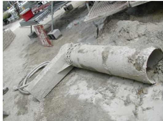
Photo courtesy of K&K Well Drilling - Batavia
