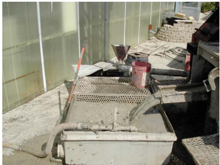
Photo courtesy of K&K Well Drilling - Batavia
