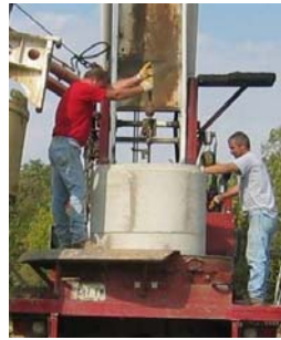
setting casing through the ring gear
