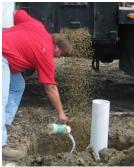
adding pea gravel & chlorine
